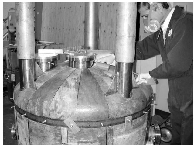
Fig. 189. Lead sheets being installed on the bottom of the ED1 tank.
