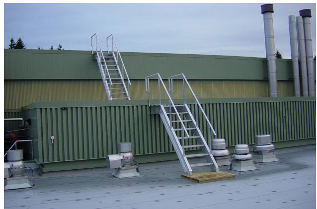
Fig. 243. The new aluminum roof access stairs (before and after).
