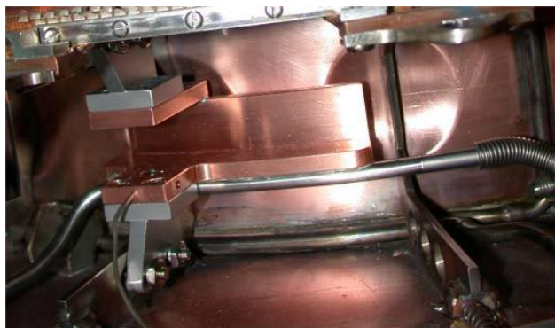
Fig. 186. Cooled beam absorber installed in Q1.
