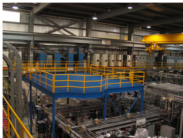
Fig. 158. Photograph of the recently installed TITAN platform in the low-energy ISAC area.
