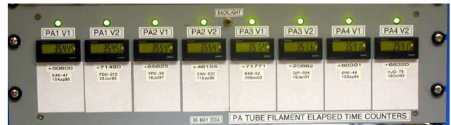
Fig. 186. New PA filament elapsed time counters.
