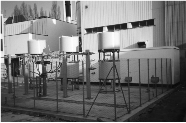
Fig. 159. Static VAR compensator for transient suppression made by GEC Alsthom, UK (40% Canadian content).
