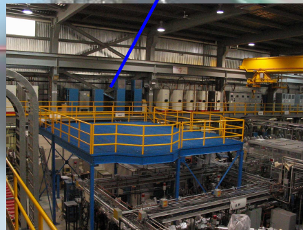
TITAN platform finished at ISAC
