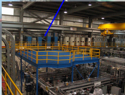
TITAN platform finished at ISAC
